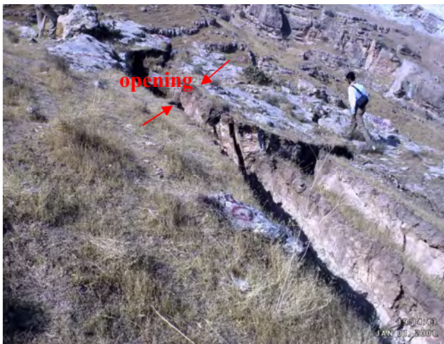
Fig. 9. The appearance of vertical joints in the southern wall of affected area and on the ground surface
