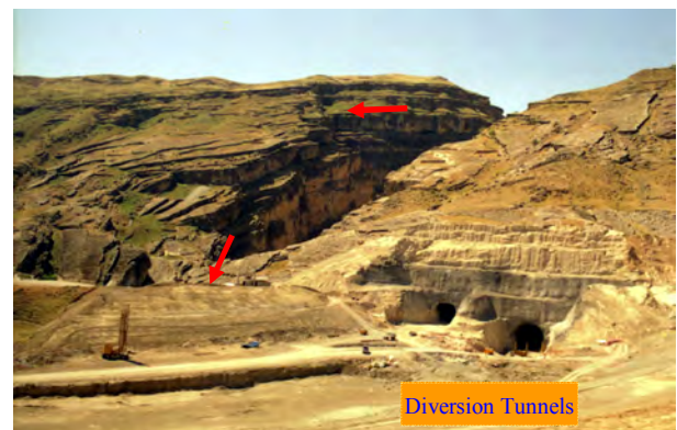
Fig. 5. Dramatic variation of bedding dips at the northern limb of Ravandi anticline
