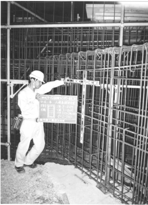
Fig. 32. Large grade beam for 14 storey building.
