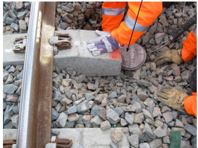
Fig. 30. Installation of pressure cells involves removing and backfilling the ballast.
