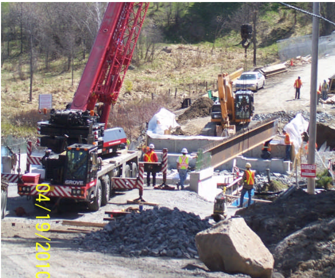
Fig.8. Bridge Girders Being Installed
