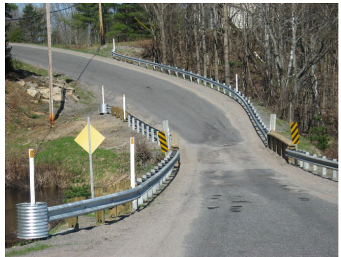
Fig.6. Existing Bridge Looking West
