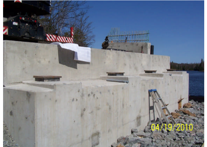
Fig.10. Completed Abutment and Bridge Seat
