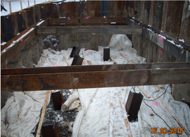
Fig.7. Installation of Abutment Piles some with Reverse Batter
