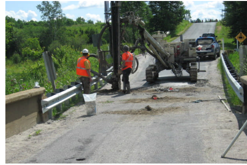
Fig.3. Air Track Rig Drilling Probe/Boreholes
