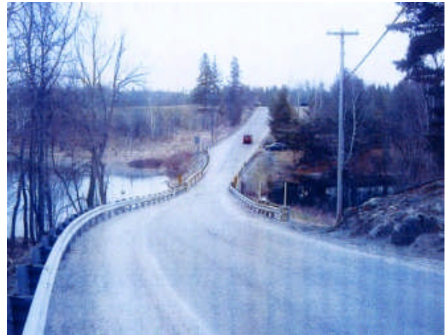
Fig.5. Existing Bridge Looking East
