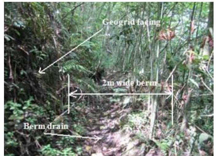
Fig.18. Photo at first berm taken on September 11, 2012 shows the site was covered with thick vegetation
