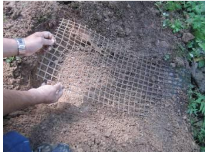
Fig.21. Sampling of buried geogrid from top layer of geogrid embankment
