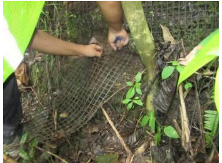
Fig. 22. Sampling of exposed geogrid from the facing
