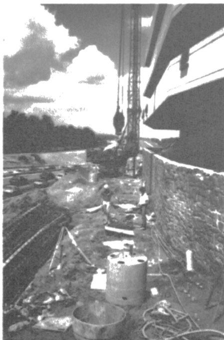
FIGURE 4. CAISSON DRILLING
