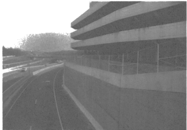
FIGURE 9. COMPLETED RETAINING WALL
