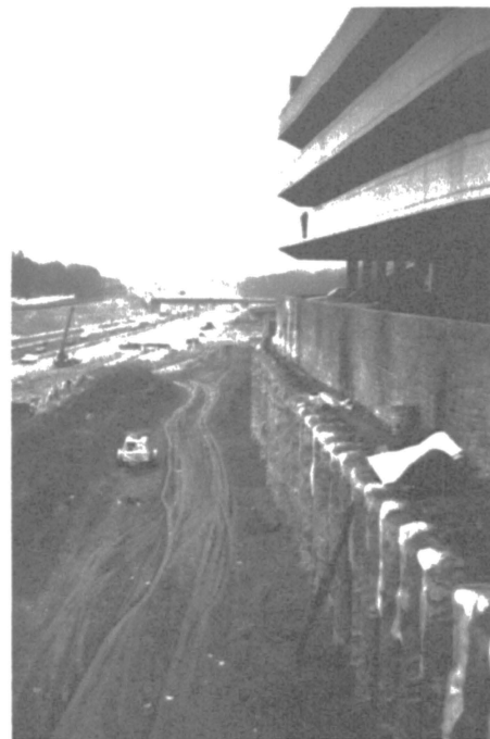
FIGURE 6. EXCAVATION IN FRONT OF WALL
