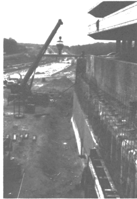
FIGURE 8. CONSTRUCTION OF CONCRETE FACING
