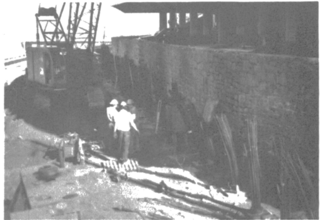
FIGURE 5. ROCK ANCHOR TENDONS
