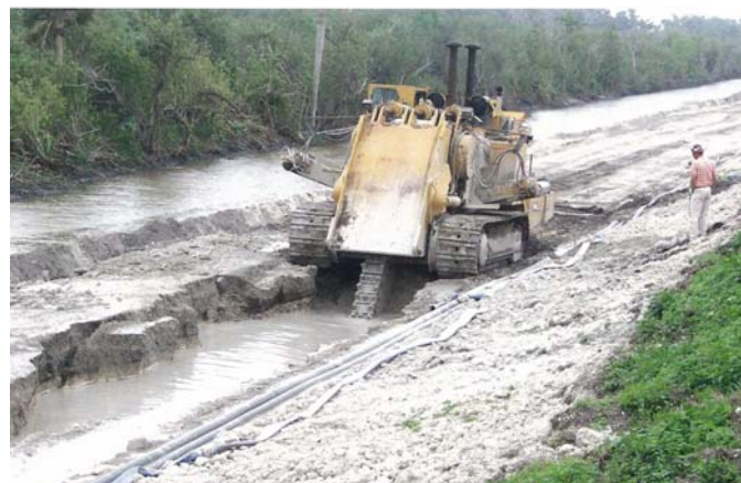
Fig. 3. Long Reach Excavator (by Others)
