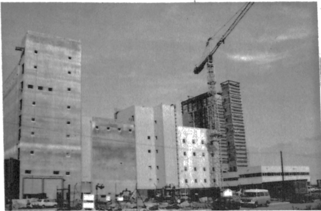
Fig. 1. Photograph of completed mill complex.
