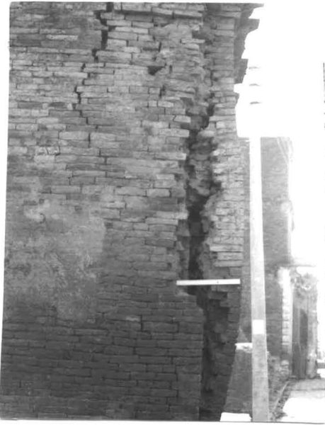
Fig. 2 Collapsing Wall
