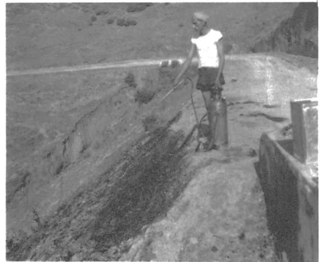
Fig. 4: Spraying of Bituminous Emulsion on the Slope.
