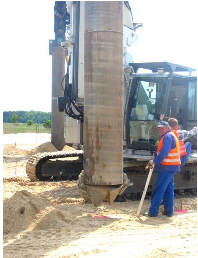
Fig. 6: In situ installation of granular soil columns
