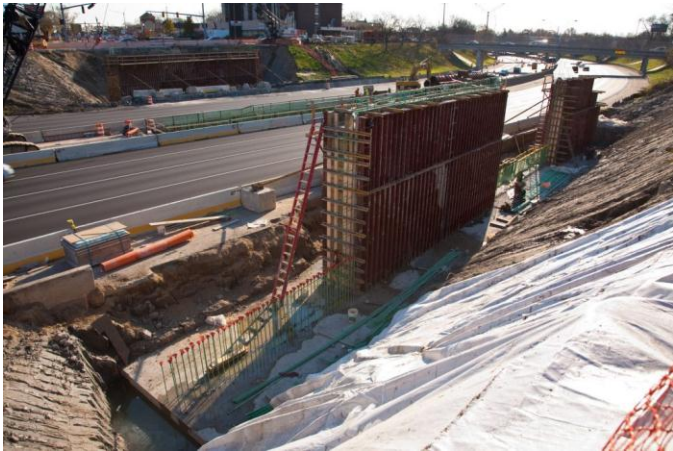
Fig. 3 West Abutment Footing and Wall
