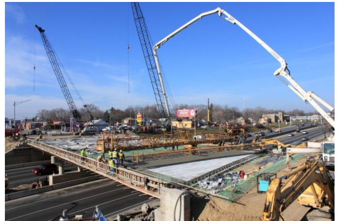
Fig. 6 Bridge Deck Under Construction
