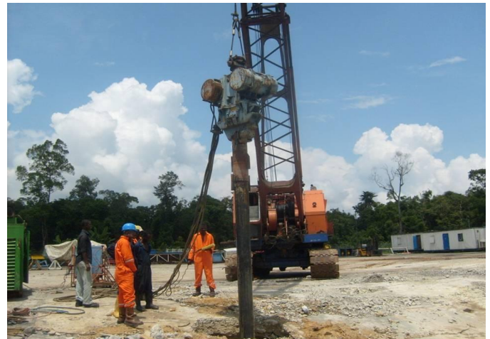
Fig. 9. Picture showing extraction of pile.
