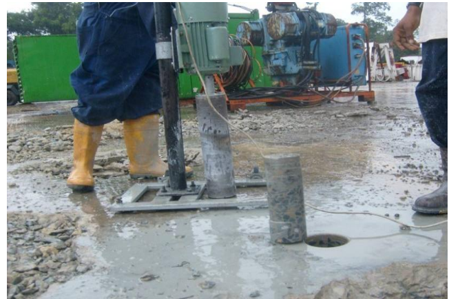
Fig. 8. Picture Showing sample after coring
