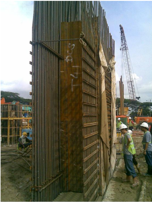
Fig. 13. Reinforcement for a female panel
