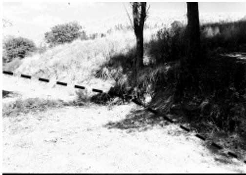
Fig. 2. Scarp above the well 6, has been caused at Manjil & Roudbar earthquake [5].
