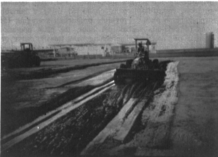
Figure 2: Grader producing cold-mix EPA via the windrowing process.
