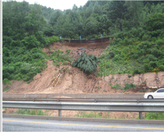
Fig 8. Picture of arc type failure
