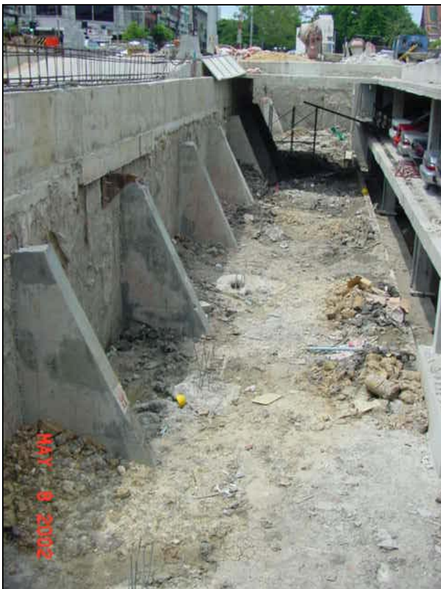
Fig. 17. View of buttress-support diaphragm wall after removal of temporary bracing
