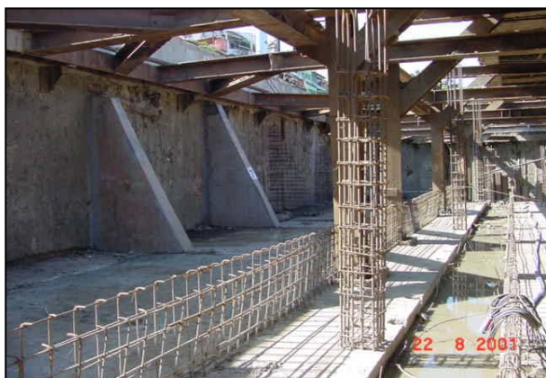
Fig. 13. View of buttress-support diaphragm wall prior to temporary bracing removal
