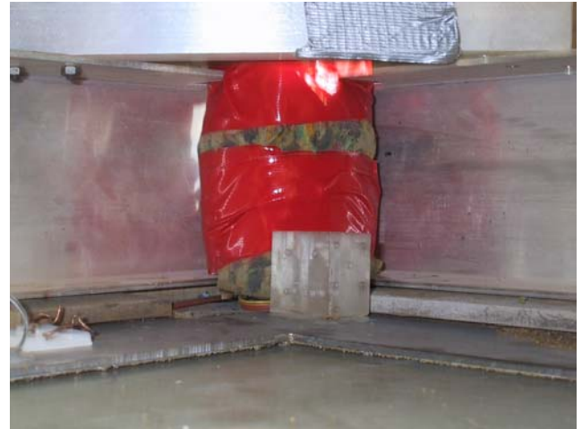
Fig. 8. The S7 accelerometer put on the foundation.
