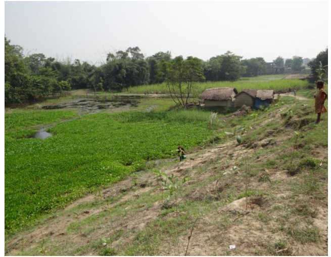
Photo 1. Lack of grass cover and intentional planting of trees on the levee side slopes
