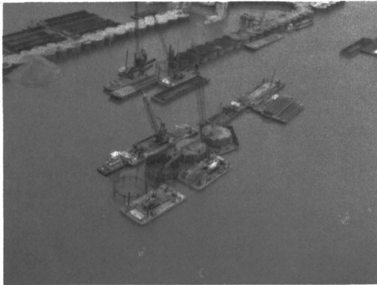
Fig. 4 Local Deflector for Cell Construction
