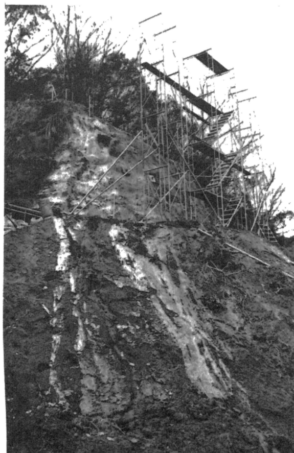
Photo 3 General View of the Field Test
