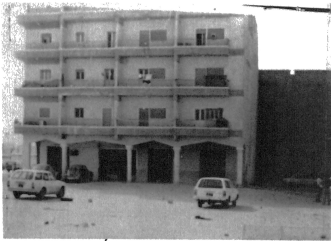
Fig.2. Front view of the Building.
