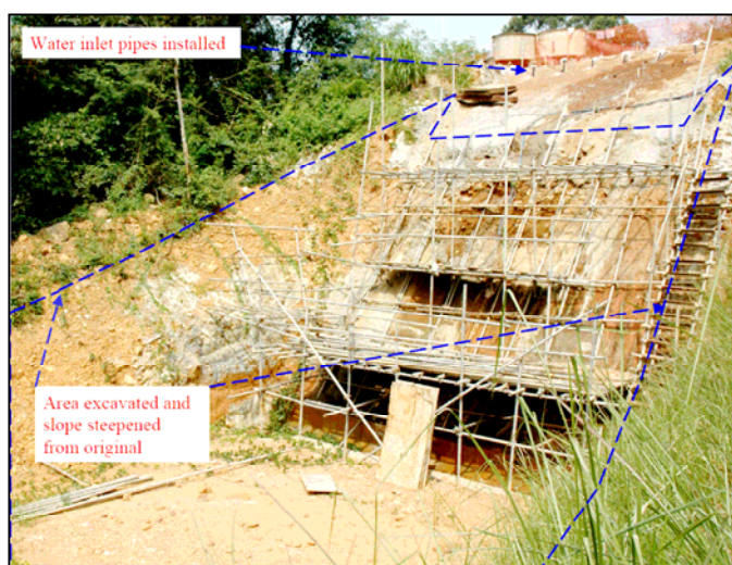
Figure 3. Overall view of slope after excavation.
