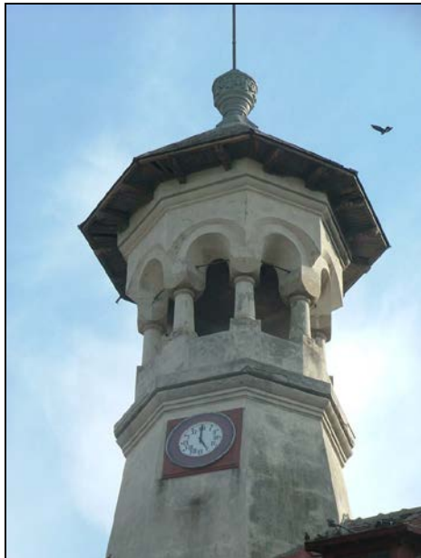
Fig. 6. Detail of the reinforced concrete turret.
