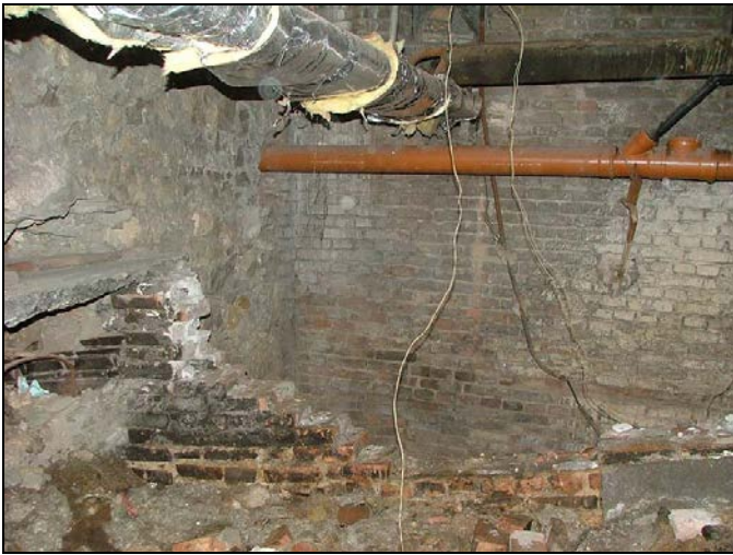
Fig. 10. View of the basement of MINA building.
