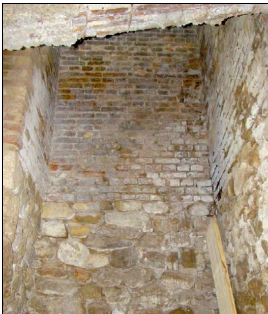
Fig. 11. MINA building: structure of foundation.
