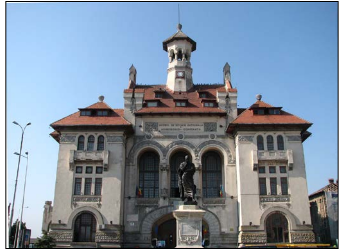
Fig. 5. General view of the main façade of the building.
