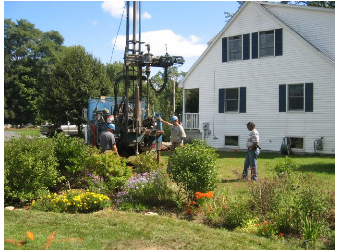
Fig.5. Test Drilling Between Adjacent Houses.
