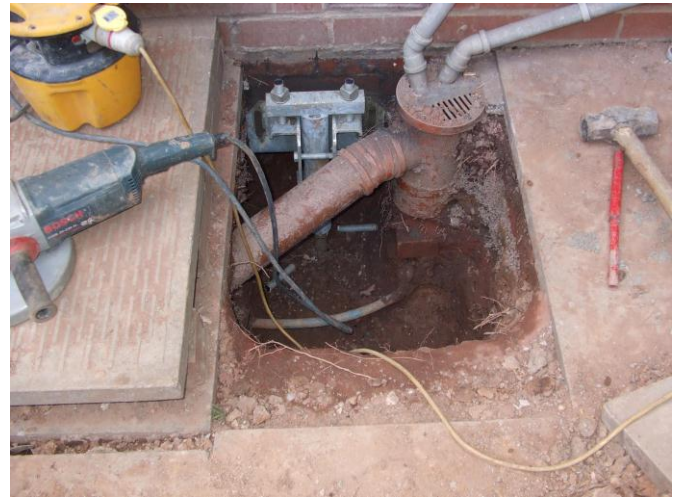
Fig. 11. Installation of a Screw-Pile Adjacent to Existing Drain Line.
