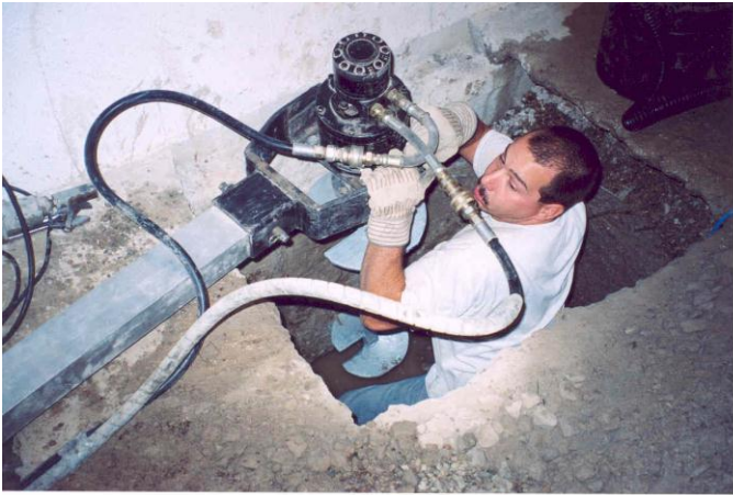
Fig. 10. Installation of a Screw-Pile Through a Cutout in a Basement Floor.
