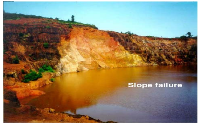
Pit Slope failure: Gross instability of benches
