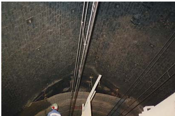
Fig. 9: Installation of the wire mesh
