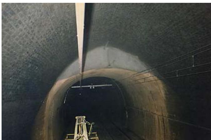
Fig. 11: Completed reinforced tunnel section
