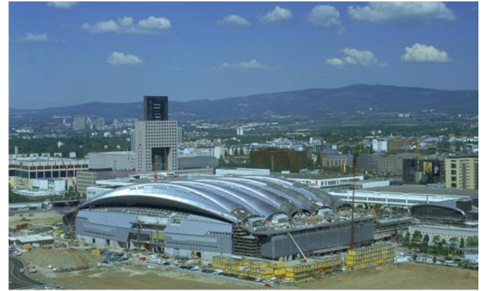
Fig. 3. New exhibition hall 3 in Frankfurt am Main
