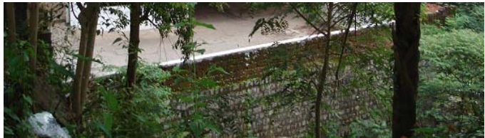
Fig. 10. Gravity masonry retaining wall
