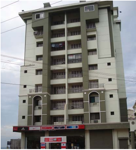
Fig. 5 RCC framed building in difficult terrain
