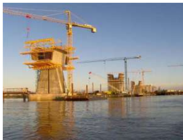
Fig. 49. General view of the construction works (courtesy of Perry da Câmara)
