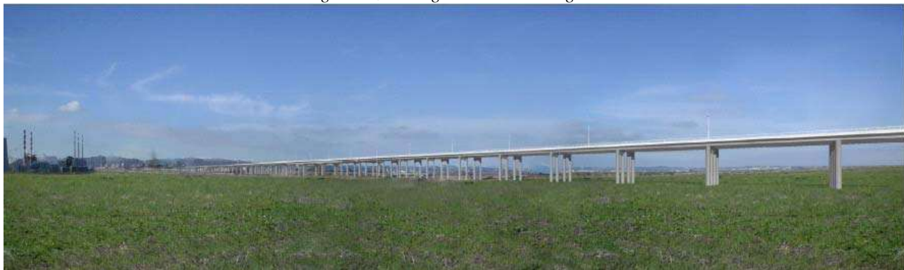
Fig. 2. North Viaduct (courtesy of Charles Lavigne )
