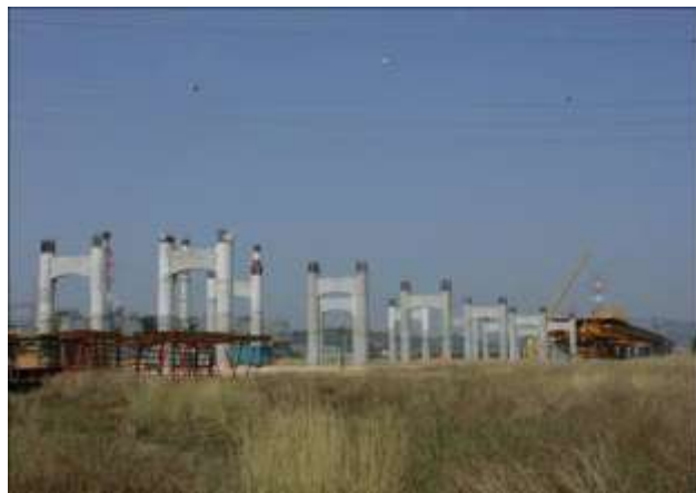
Fig. 41. Construction of North Viaduct
