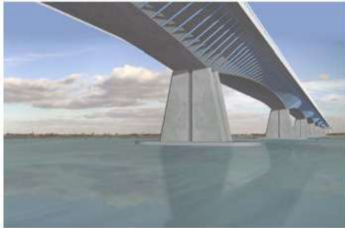
Fig. 3. Main Bridge (courtesy of Charles Lavigne)
