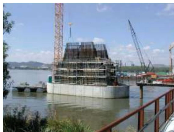
Fig. 48. Pier under construction (courtesy of Perry da Câmara)
