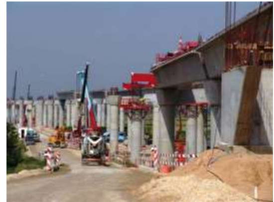
Fig. 43. Construction of South Viaduct
