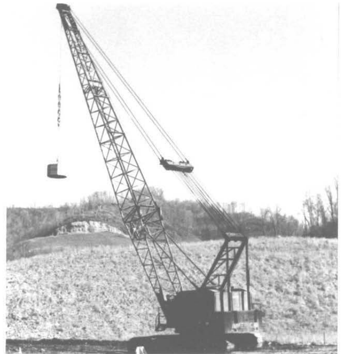
Fig. 3 - Crane lifting a 15-ton weight 70 ft
