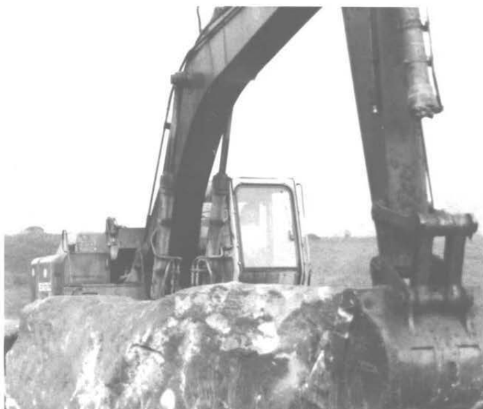
Fig. 2 - Large boulder excavated from test pit
