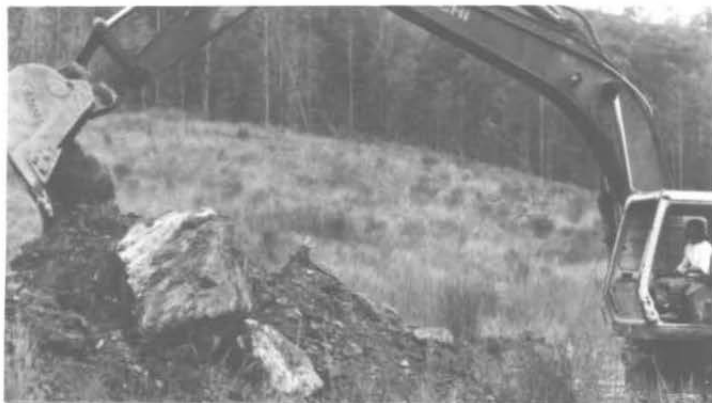
Fig. 1 - Typical mine spoil fill
