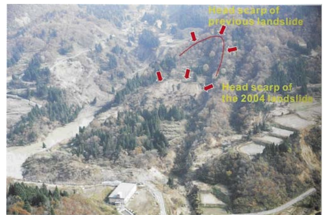
Fig. 6. The Higashi-Takezawa landslide (source: Sassa et al, 2005)
