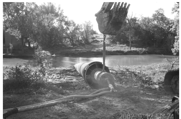
Fig. 10. Photo showing 60-inch casing installation.
