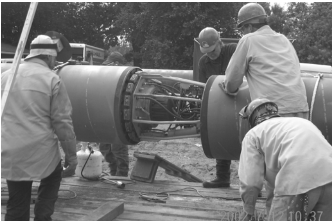
Fig. 7. Photo showing pipe assembly.
