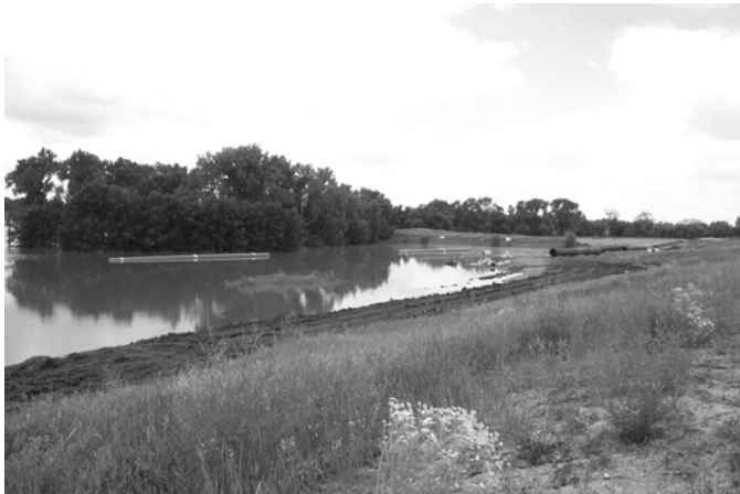
Fig. 3. Photo showing flooded staging area.
