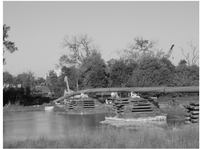
Fig. 8. Photo showing float used to support pipe during pull.
