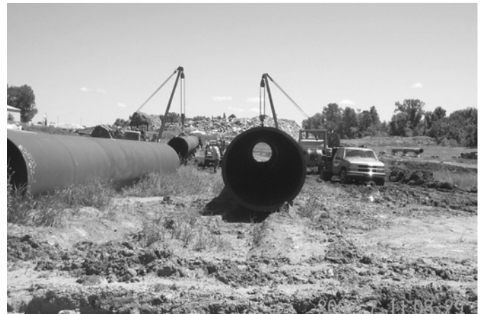
Fig. 9. Photo showing 60-inch casing assembly.
