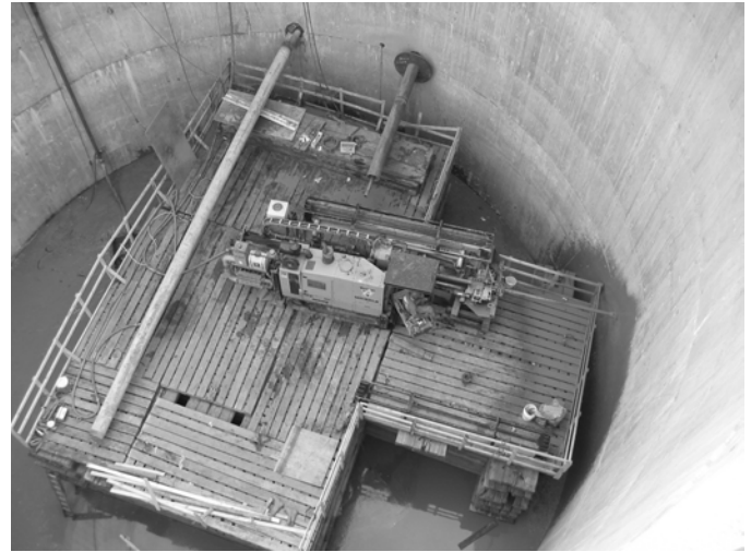
Fig. 4. Photo showing drilling pilot to drill rig.
