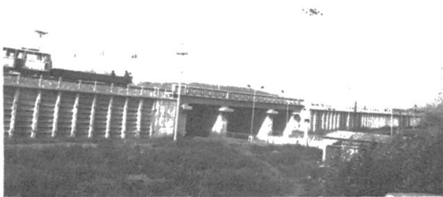
Fig. 1. The Whole Scene of Ba-Yu-Quan Anchor Slab Retaining Wall
