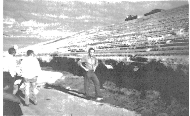
Figure 3. - Exposed embankment behind soil-cement at Cheney Dam.
