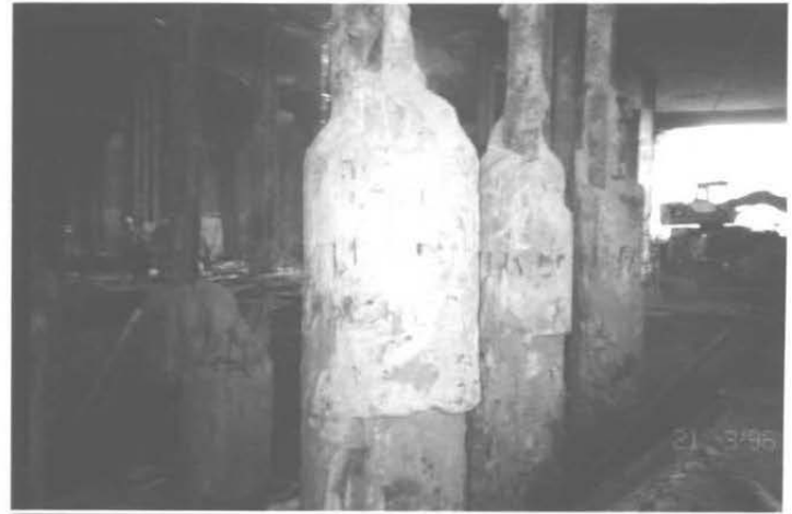
Fig. 6 The photograph illustrates the pile size changes caused by difference in diameter of temporary casing and auger used in pile construction.
