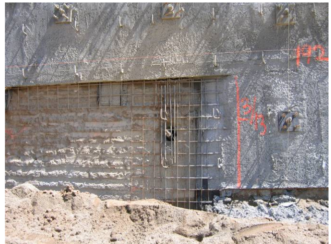
Fig. 1. Soil nail retaining wall during construction
