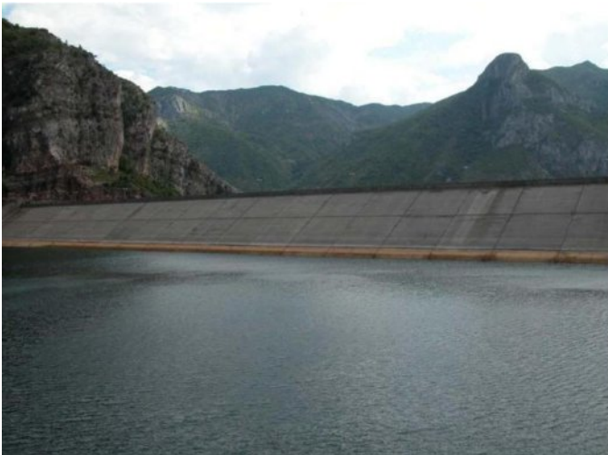
Fig. 2: Koman dam – upstream view
