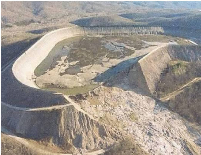
Fig. 3. Breach through Taum Sauk embankment
