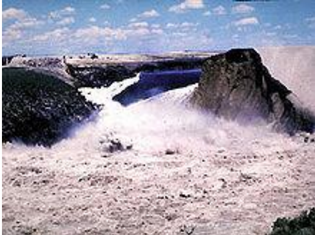
Fig. 4. The Teton dam after failure.
