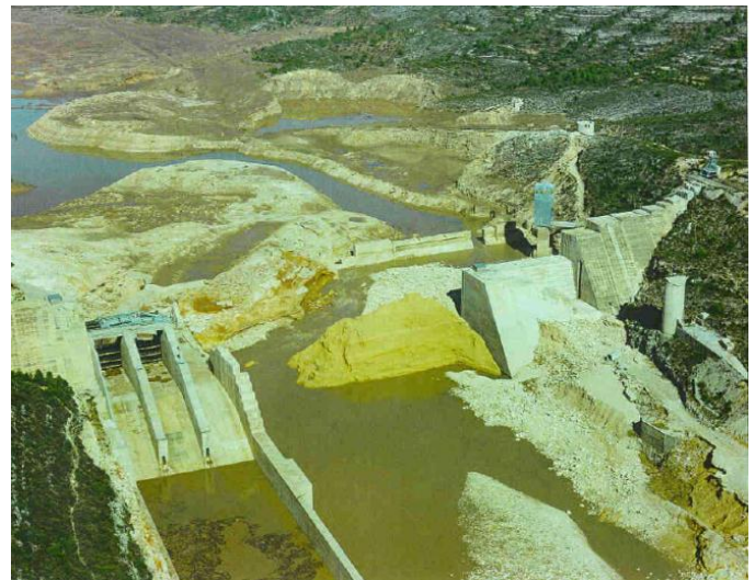
Fig. 2. The Tous dam after failure.
