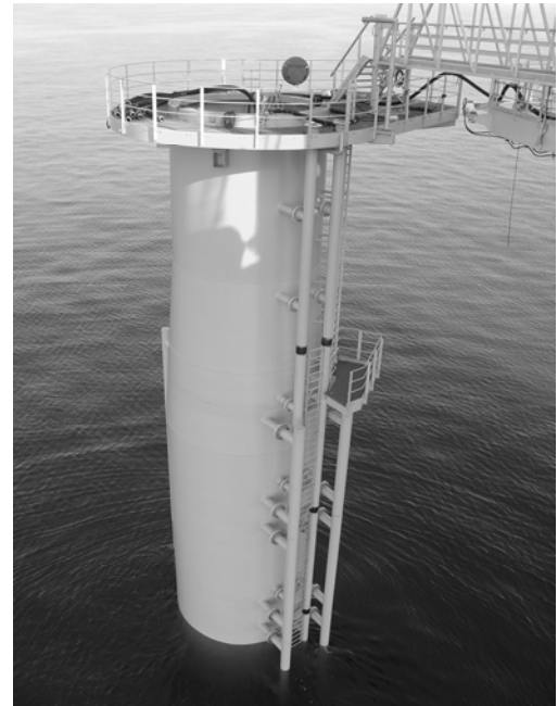
Fig. 6. Transition piece
