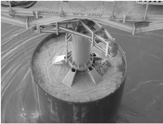
Fig. 19. Flydrill BFD 5500 with KB3000 just before exiting pile
