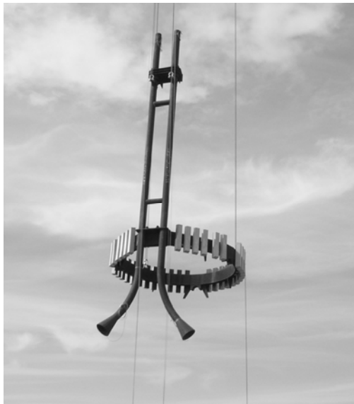
Fig. 4. J-tube and anode ring
