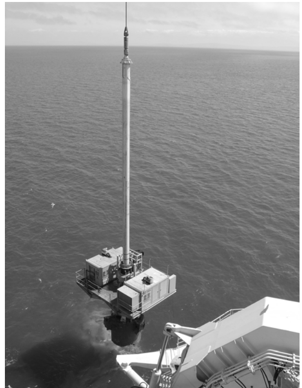
Fig. 15. Flydrill BFD 5500 with KB 4400 reaming bucket
