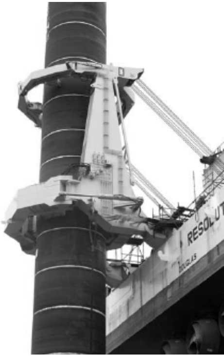
Fig. 12. Upended' monopile (Reproduced by kind permission of Gusto B.V. Holland)
