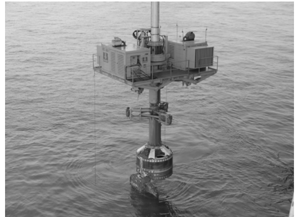
Fig. 21. KB 3000 Pre-bore bucket just above sea level
