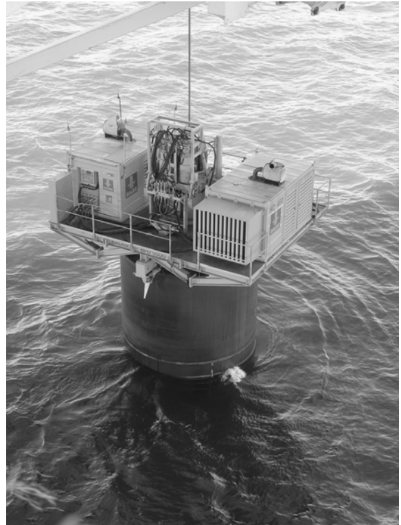
Fig. 18. Flydrill BFD 5500 drilling on top of a monopile
