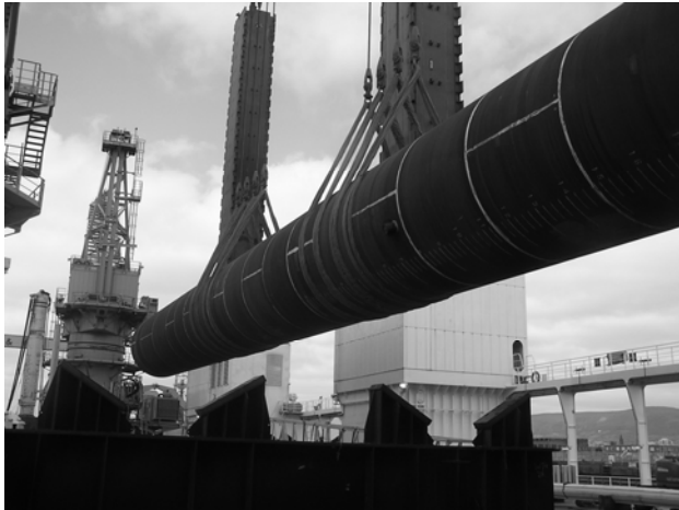
Fig. 8. Monopile being lifted into position
