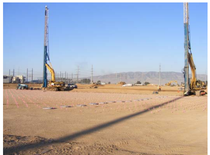
Fig. 4. Wick Drain Installation
