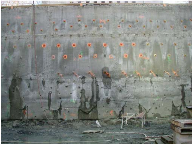
Fig. 1. Photograph of east wall during construction.
