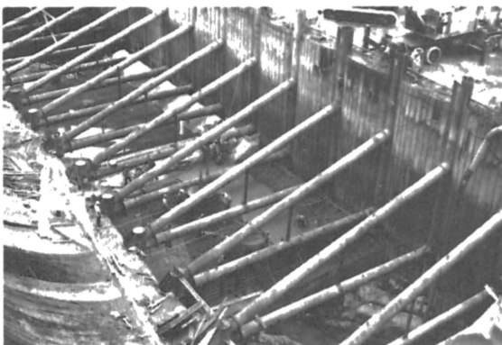
Fig. 4. Completed Cofferdam
