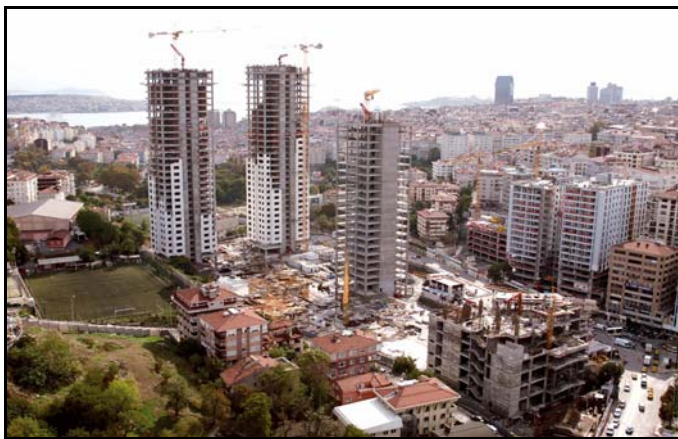
Fig.4. BJK Fulya Complex - during the construction, September 2007
