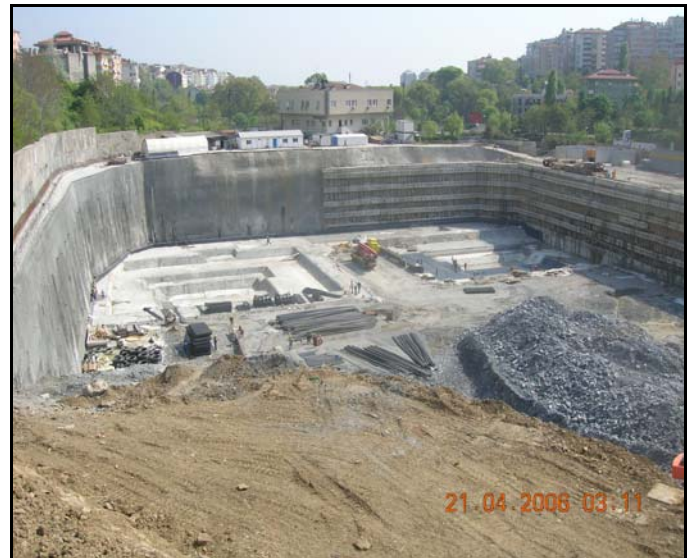
Fig.13a. Retaining system facing north side
