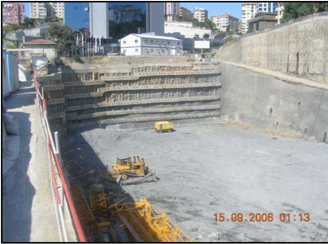
Fig.13b. Retaining system facing south side
