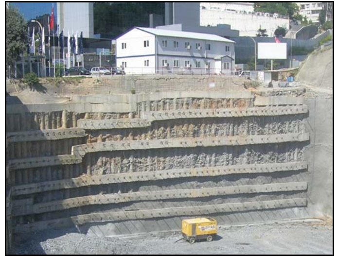
Fig. 12d. Reinforced concrete walls under the bored piles
