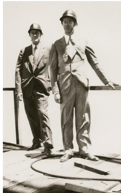
Fig. 10. Ralph and Orwin Peck standing atop the north tower of the Golden Gate Bridge on July 30, 1936, while it was under construction. This was a special honor not accorded to very many visitors. Note early model "boiled" hard hats (Peck family).
