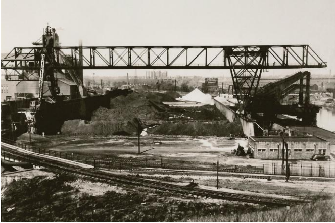
Fig. 46. Ore Storage Yard at Republic Steel's Blast Furnace No. 5 in Cleveland, where Terzaghi made a grievous error in settlement calculations. If it hadn't been caught by Peck, the ore piles to have been stacked so high they would have suffered bearing capacity failures (Peck Collection-NGI).
