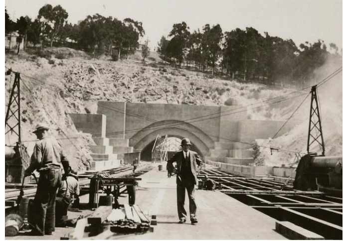
Fig 9. Ralph standing on the west tail span of the Oakland Bay Bridge with the eastern portal of the Yerba Buena Tunnel behind him. The tunnel measured 56 feet wide with a height of 76 feet, making it the largest tunnel in the world at that time (Peck family).
