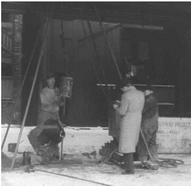
Fig. 23. Ralph Peck (in light colored jacket at middle right) logging his first boring for the Chicago Subway in February 1939 along the State Street Route (Peck Collection-NGI).
