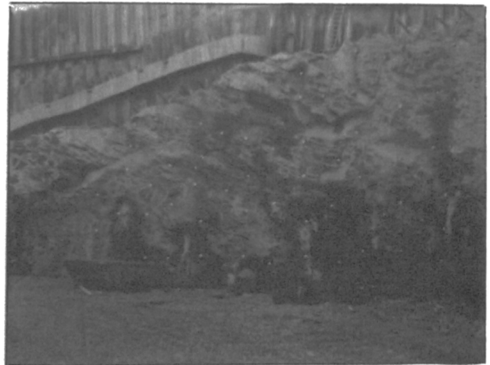
Fig. 13. Rock slope face at the final excavation line reinforced with bolts.
