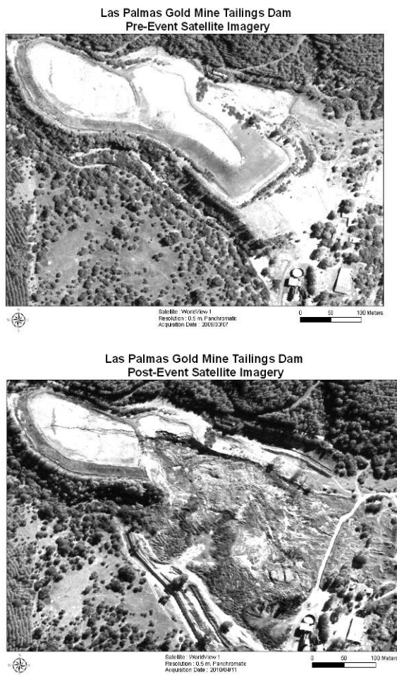
Fig. 8. Pre and post satellite images of failed tailings impoundment.
