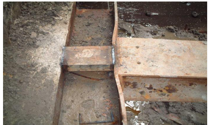
Plate 2. Photograph of Revised Stiffener
