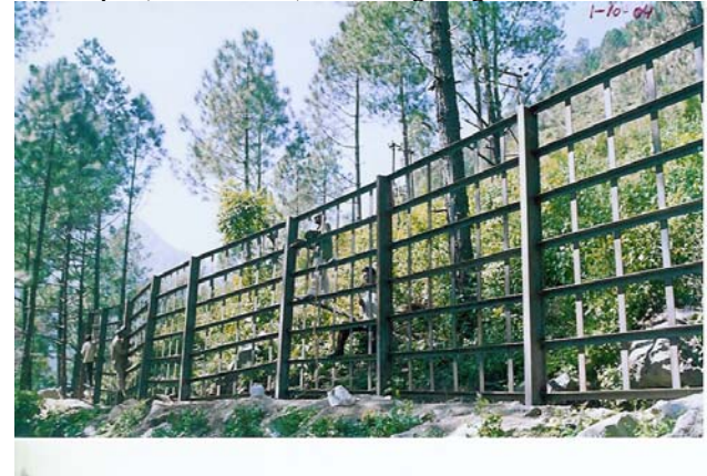
Fig.8 Restraint measures by construction of Steel barricading structure
